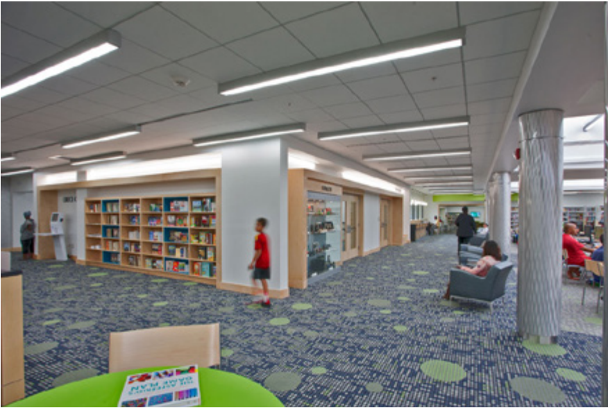
4" aperture surface mounted linear downlight with flush lens providing high angle illumination.
