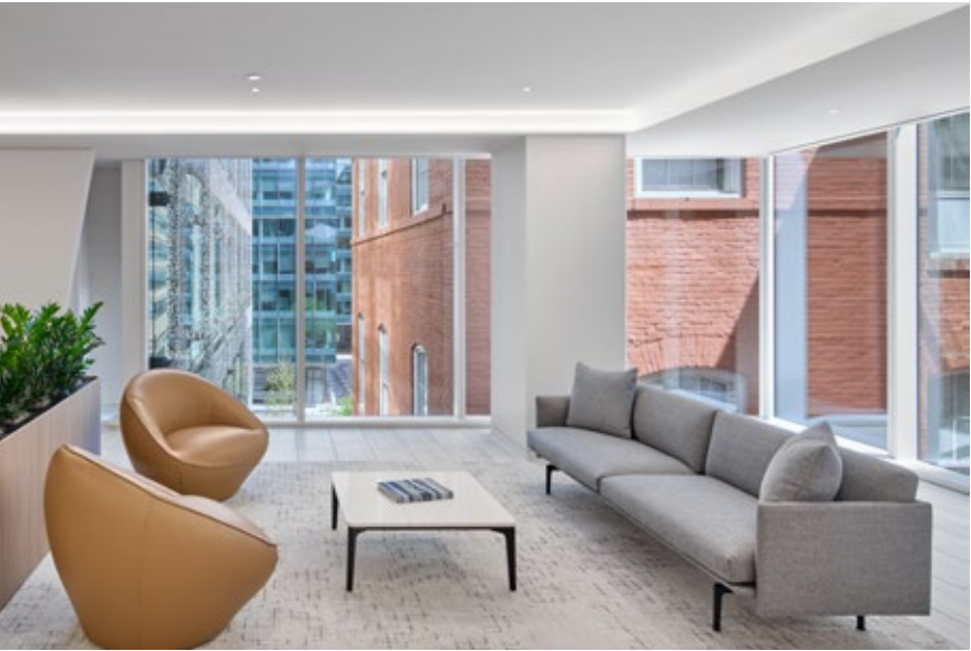
Non-illuminated cove system featuring plaster-in precision knife edge for clean, minimal effect.
