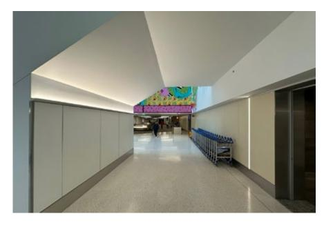
Continuous surface wall, ceiling or mullion mounted cove system that delivers an even wash of directed light to the ceiling above or the floor below, and redirected light to softly illuminate the wall behind the fixture.
